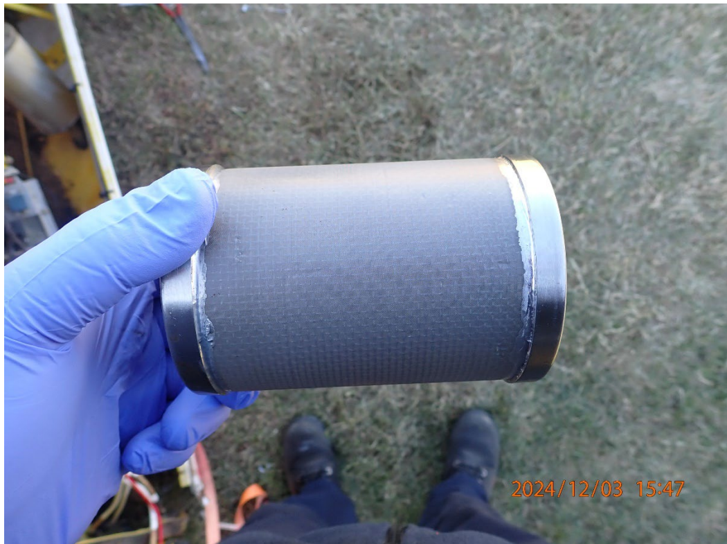
Photo 5: View of the unobstructed fuel strainer screen.
