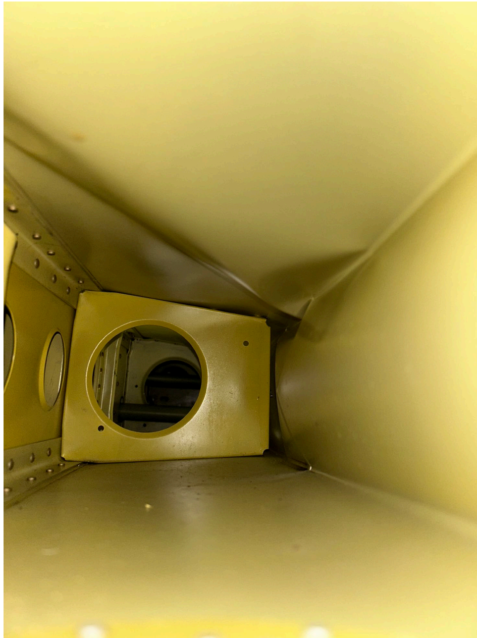
Photo 5 – Interior View of Left Wing Structure Forward of Aileron (FAA)
