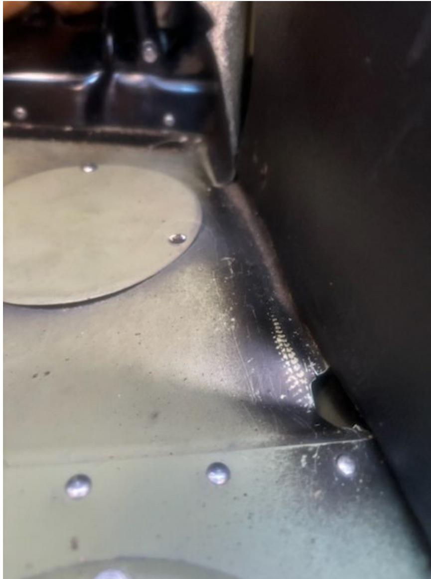
Photograph 3 - Floorboard buckling impact damage (Courtesy of FAA)
