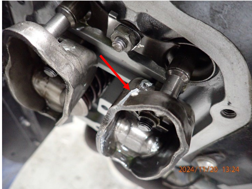
Visible Assembly Lubrication Oil Present on Rocker Arms
