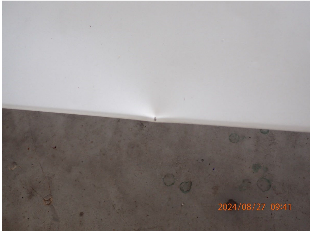
Photo 8: View of damage to the trailing edge of the right stabilator trim tab.
