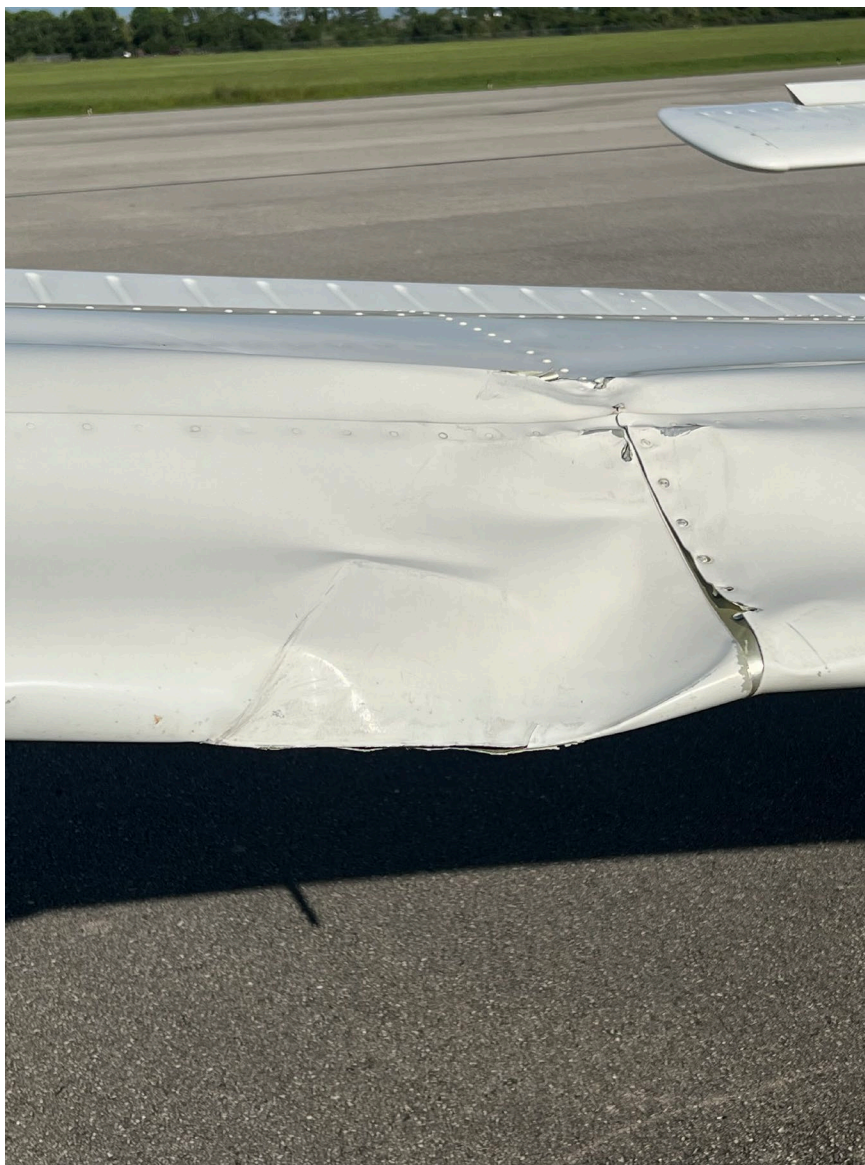
Photograph 5 - Damage to low-wing airplane's wing (Courtesy of Skyborne Airlines)
