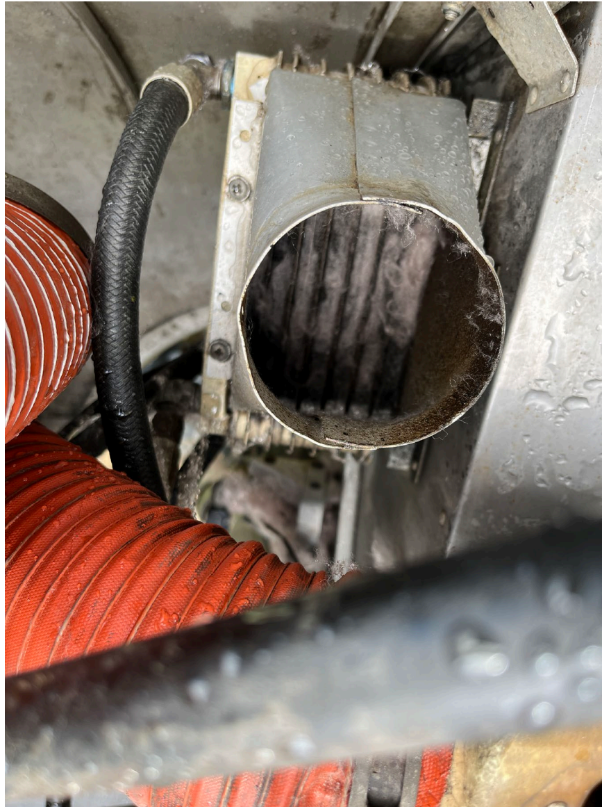
Photograph 2 - oil cooler obstructed with a residential-type insulation (Courtesy of FAA)
