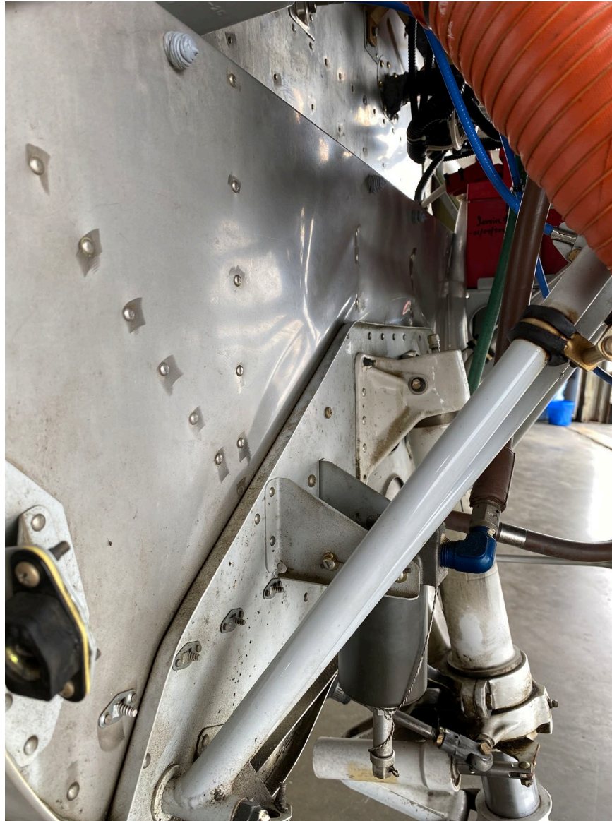
Photograph 1 - Postaccident firewall damage (Courtesy of FAA)
