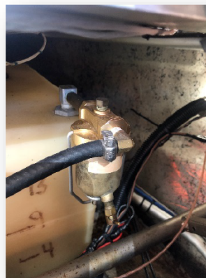
Figure 1 - Excerpt from Aventura II POH depicting fuel drain valve installation.
