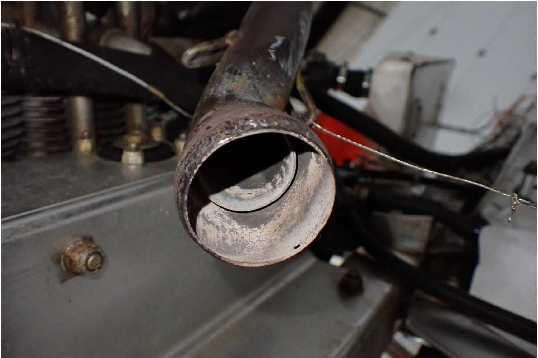
Photograph 15 - No. 4 exhaust riser end
