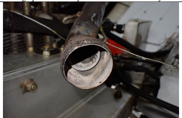
Photograph 31: No. 4 cylinder exhaust riser end
