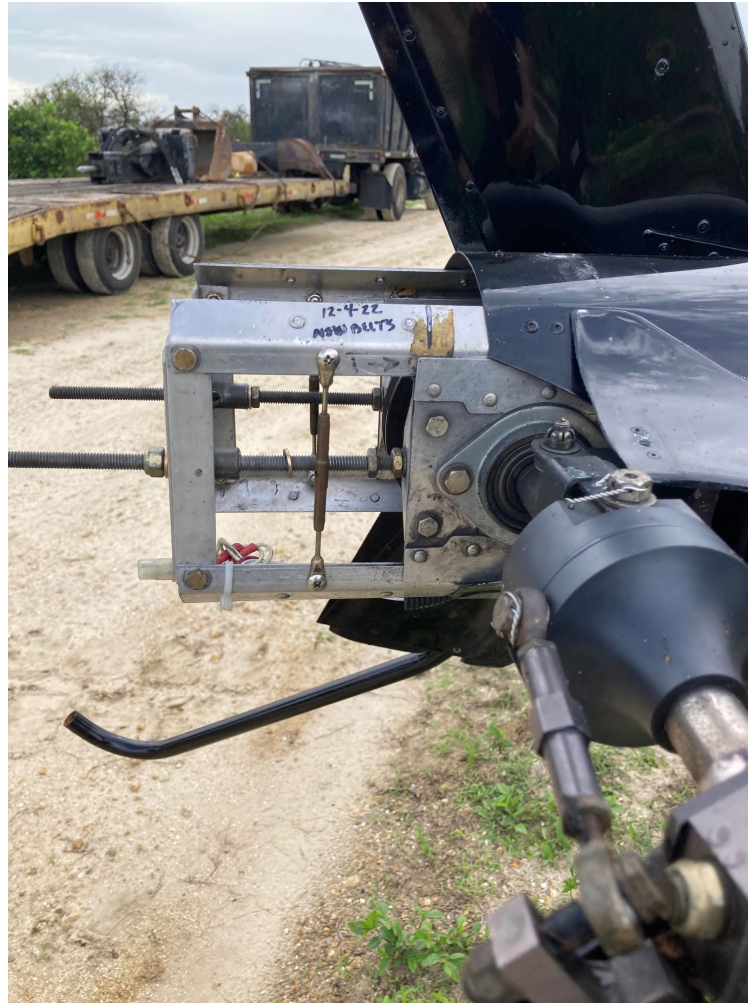
Photograph 4 - Side view of the tail rotor drive belt jam nut out of position. (Courtesy of Pilot/Owner)
