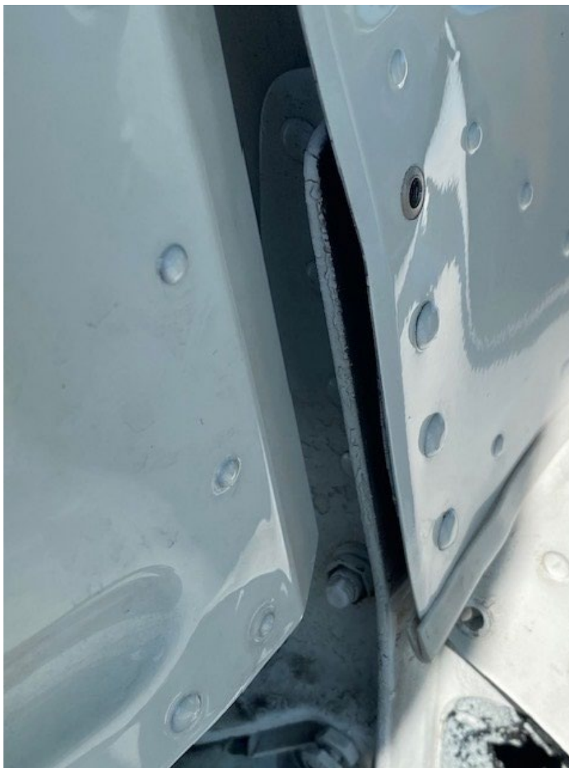
Photograph 2 - Right side Vertical stabilizer with missing rivet (Courtesy of Skyborne)
