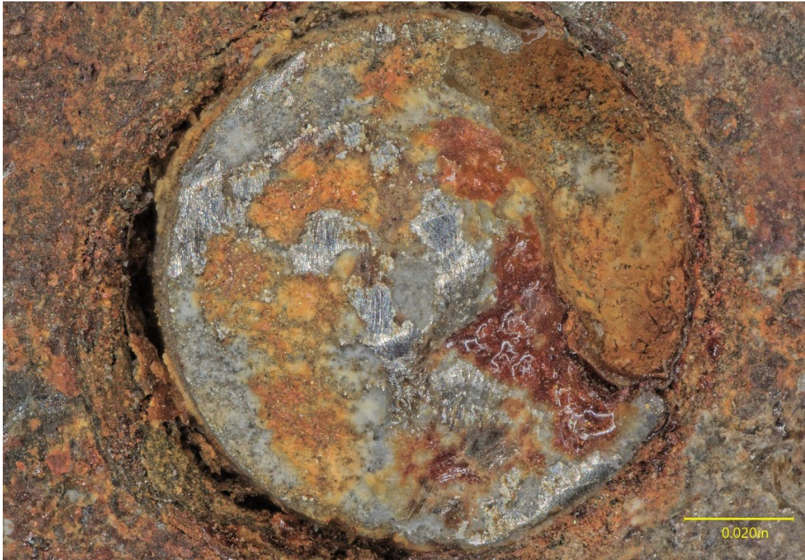
Figure 14. The lower rivet fracture surface, as received.
