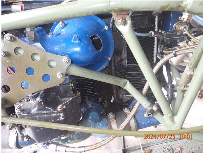
Figure 9 Carb Heat Box Damage
