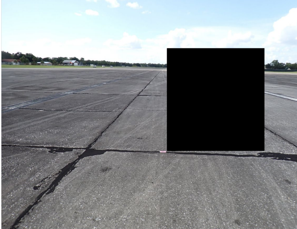
Figure 8 View of Runway in Direction of Landing With Pink Marker on Runway Showing Marks From Left Main Landing Gear Tires
