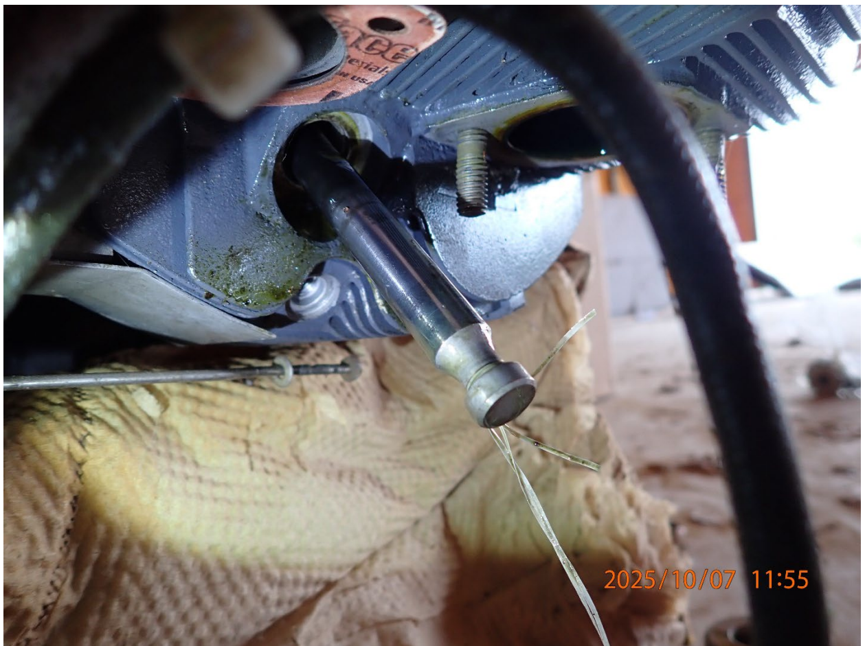
Photo 1: View of the No. 1 exhaust valve stem.
