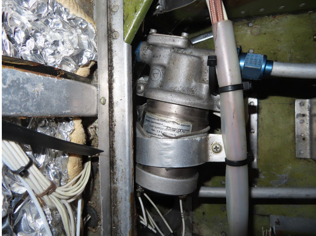
Photo 15: View of the electric fuel pump. (Piper Photo)
