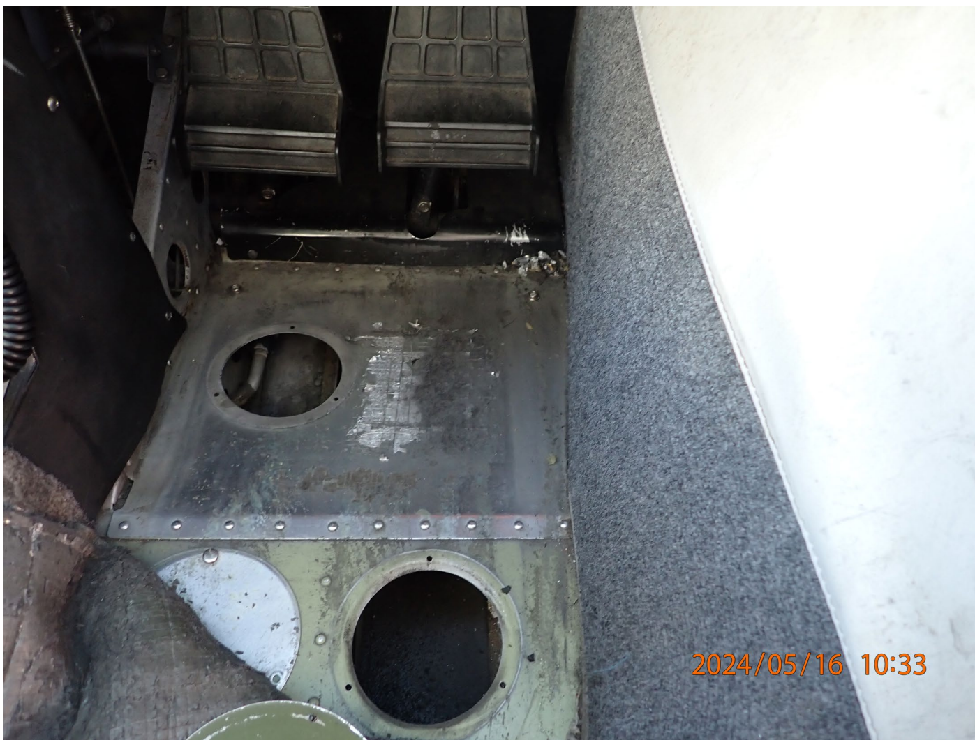
Photograph 3 - View of floor damage.
