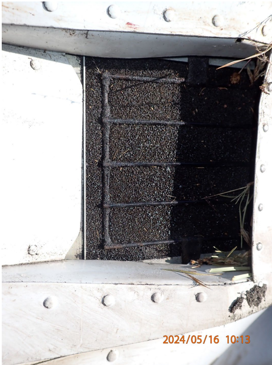
Photo 19: View of the air intake filter.
