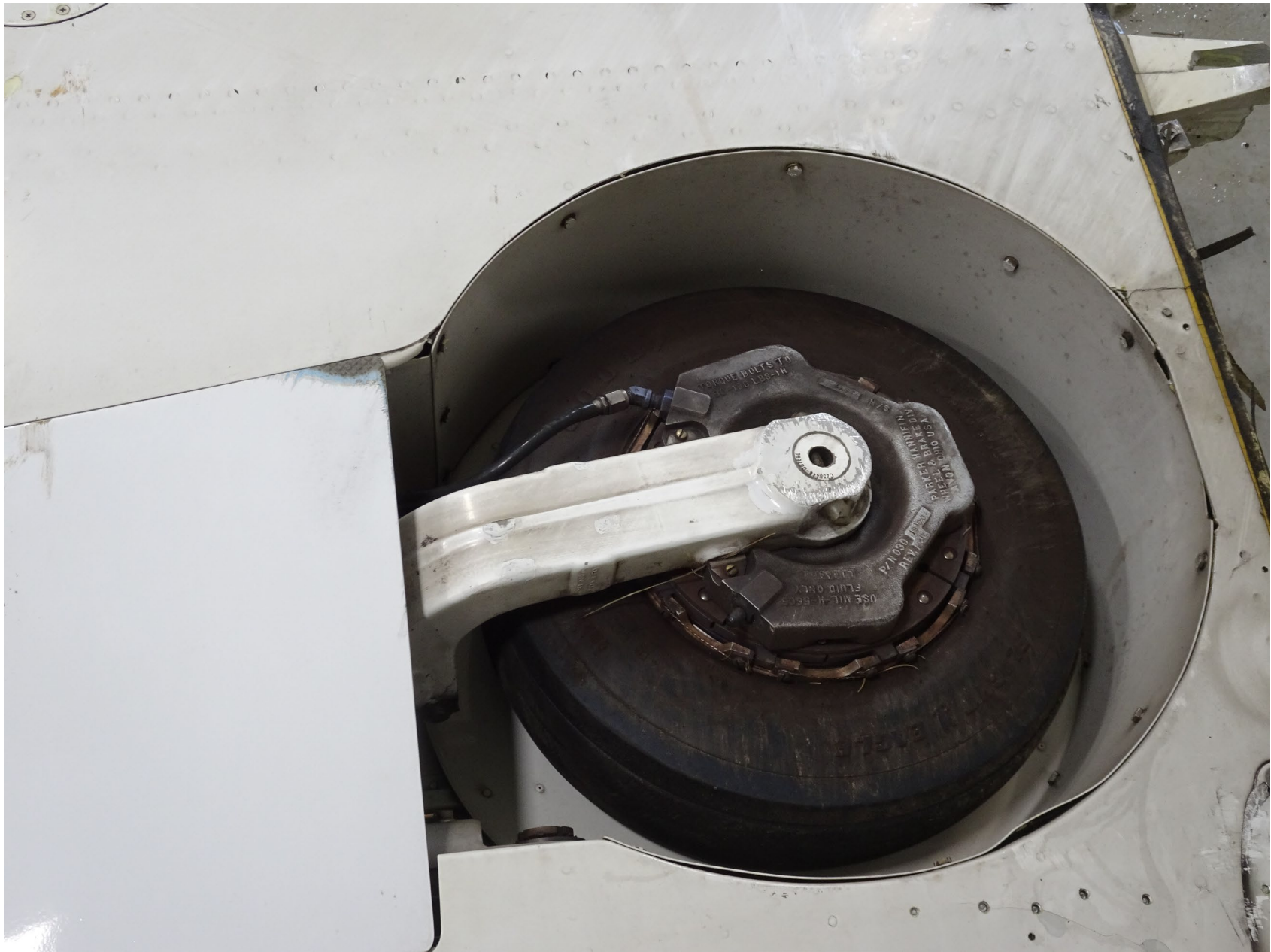
Photo 6 – View of Right Main Landing Gear as Found (RDU)
