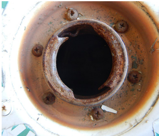
Photo 7 - View of the right fuel tank filler neck with rust.
