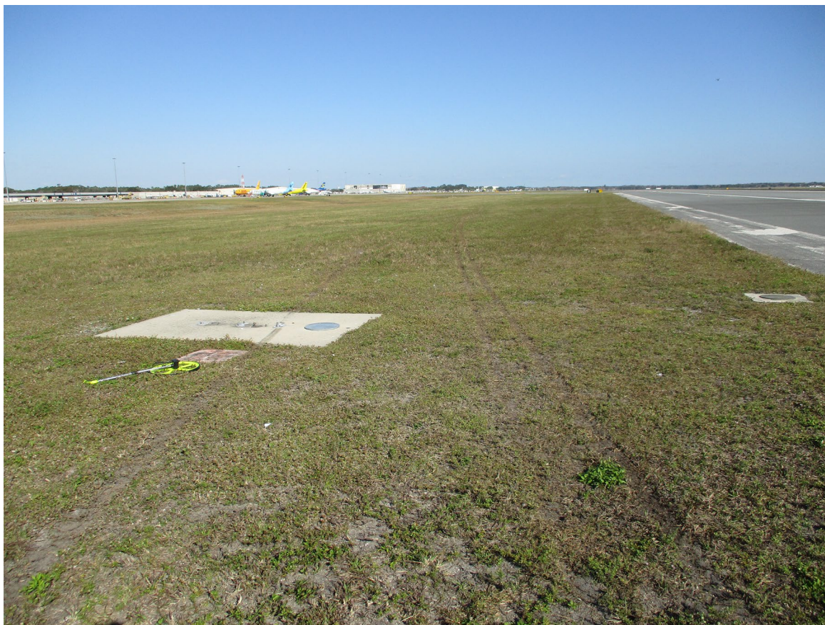
Photograph 7 - View of the Tire Marks in Grass and On Concrete Pad of Impacted Runway Marking Sign (Courtesy of FAA)
