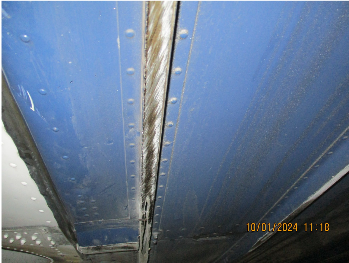
Photograph 3 - Damage to external longerons (Courtesy of FAA)
