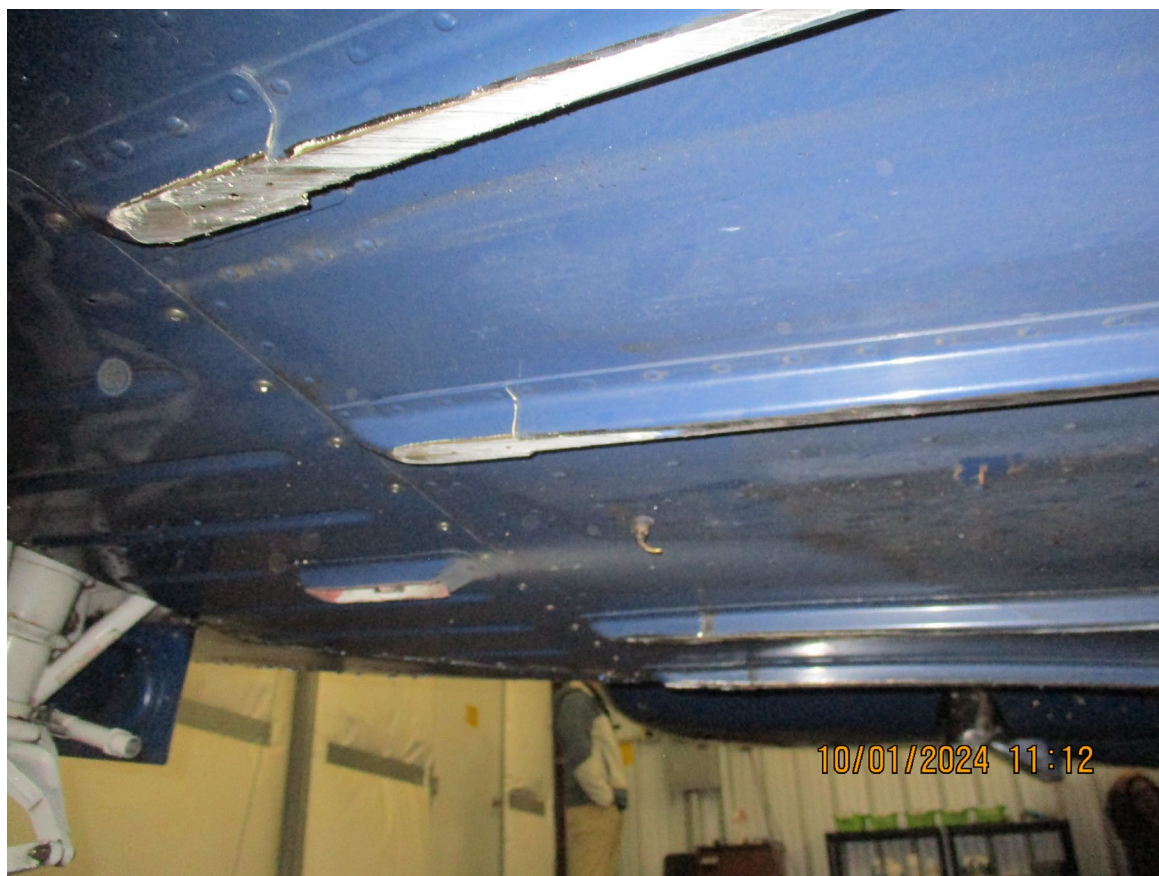
Photograph 4 - Damage to external longerons (Courtesy of FAA)
