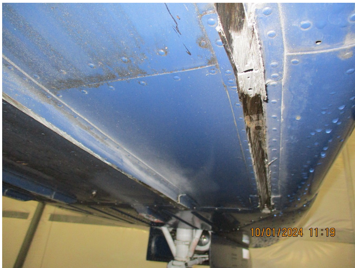
Photograph 2 - Damage to external longerons (Courtesy of FAA)
