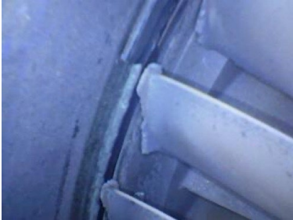
Photo 6 - Missing wheel shroud on stage four turbine wheel as viewed through the exhaust collector support via borescope.
