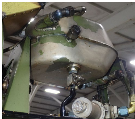
Photo 4 - View of engine oil tank.
