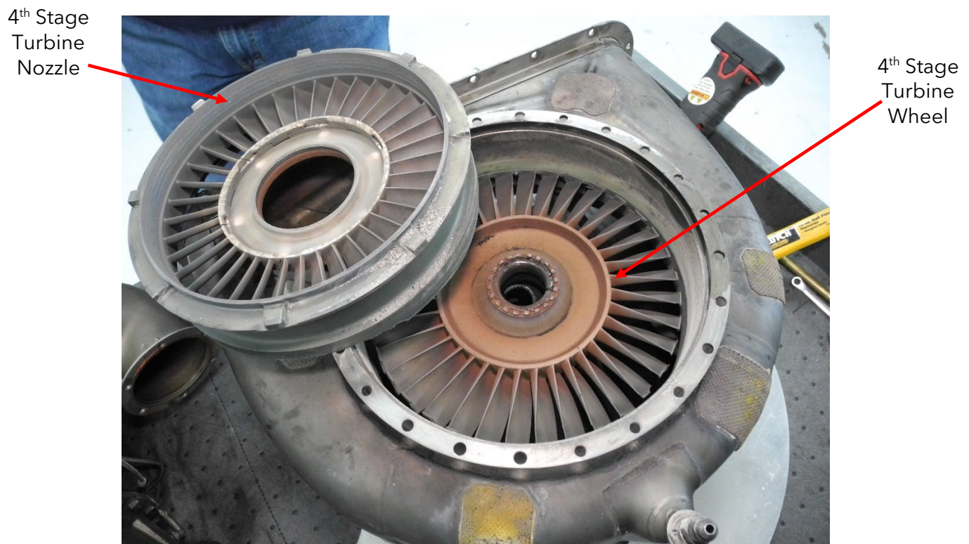
Photo 14 – 4 th Stage Nozzle and Turbine in Exhaust Collector Support Housing
