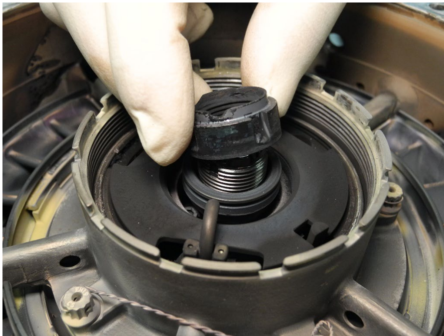
Photo 23 - No. 8 Bearing Spanner Nut - Loose
