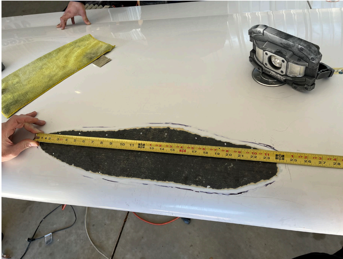
Photograph 2 - Measurement of delamination/disbonding (Courtesy of FAA)
