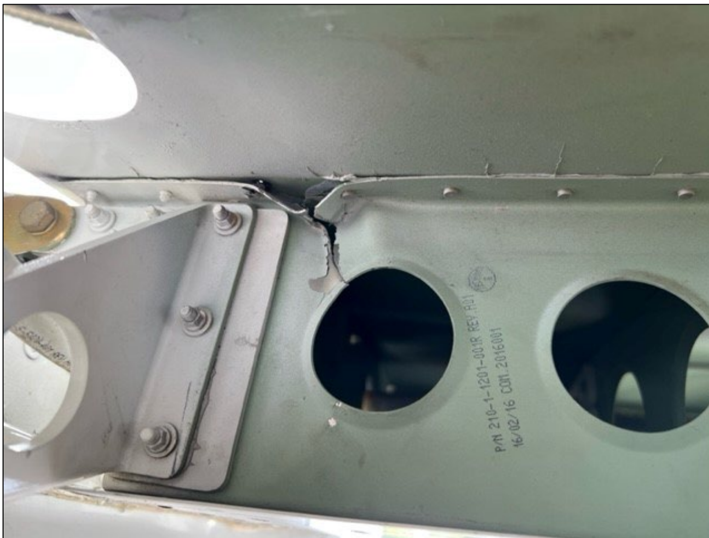
Figure 3: Internal view of the right wing damage (Photo Courtesy FAA)
