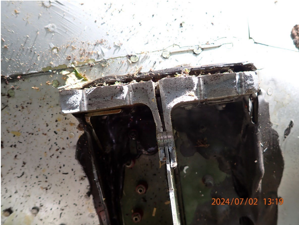
Photo 13: View of the left main wing spar.
