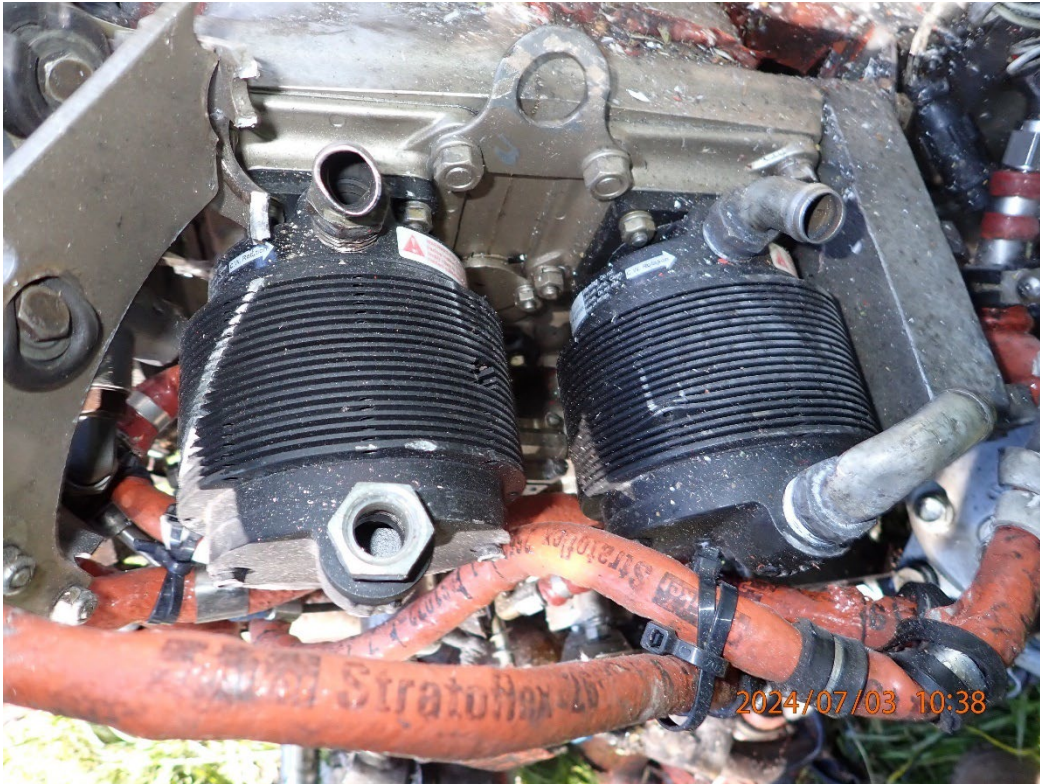
Photo 41: View of the vacuum pumps installed on the engine.
