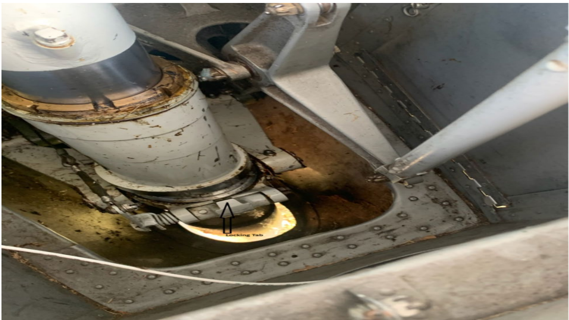
Figure 3. Picture taken by FAA inspector during onsite examination.
