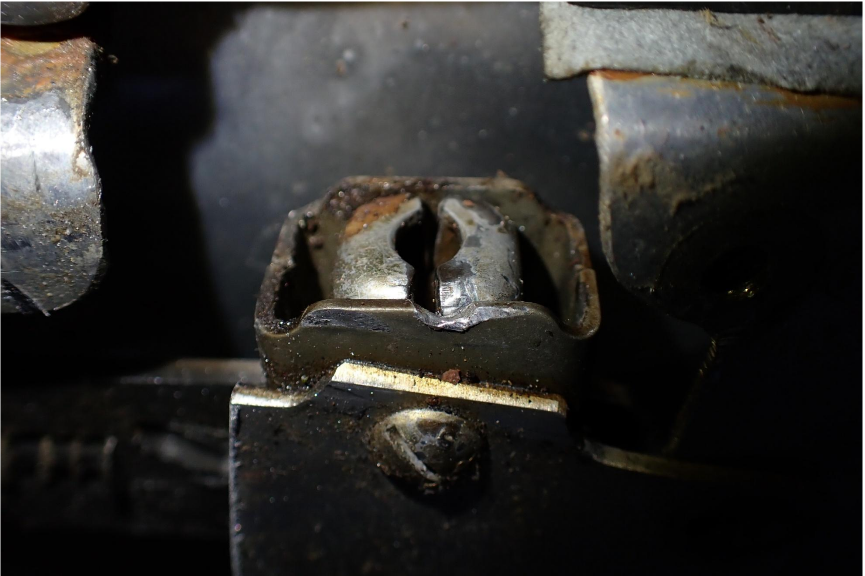
Photograph 8 - Main cabin door upper latch
