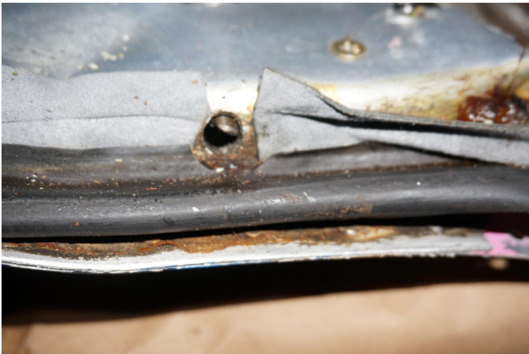
Photograph 6 - Main cabin door aft latch pin
