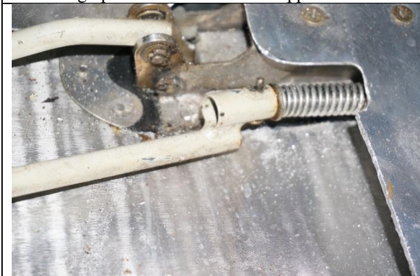
Photograph 16: Main cabin door aft door latch pin, and actuating rod
