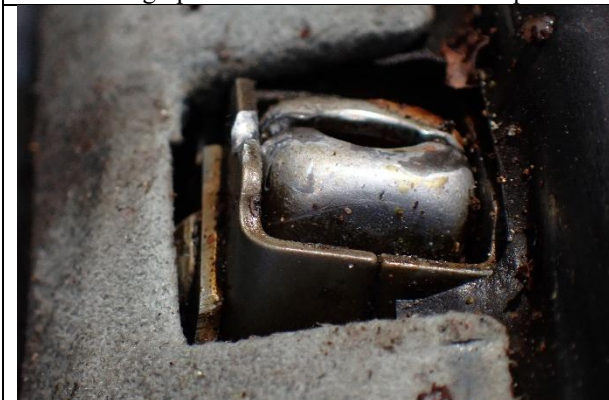
Photograph 10: Main cabin door upper door latch
