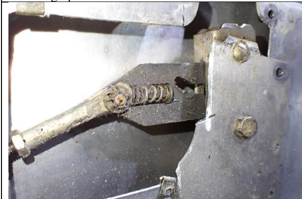
Photograph 14: Main cabin door upper door latch
