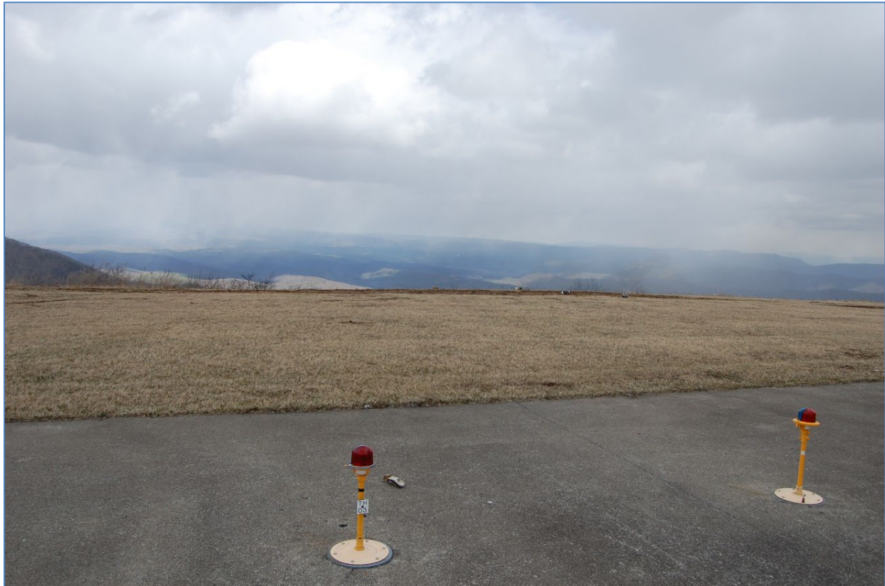
Figure 4 - Photograph at 1520 EDT looking northeast from the touchdown point of runway 25 towards the approach path to the runway after the accident.
