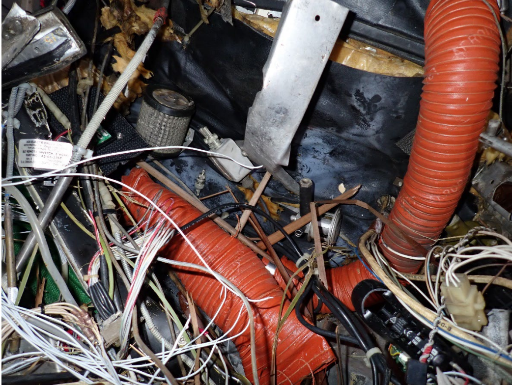
Photo 48: View of vacuum filter and relief valve. (Textron Aviation Photo)
