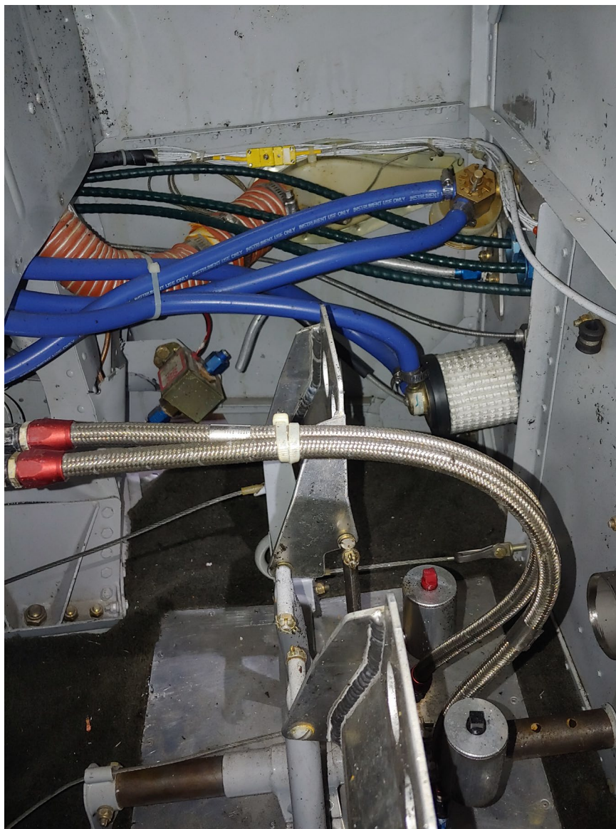
Photograph 6 - View of boost pump with fractured fuel line. (Courtesy of FAA)
