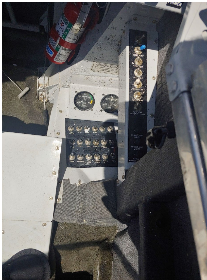
Photograph 5 - View of switches and circuit breakers. (Courtesy of FAA)
