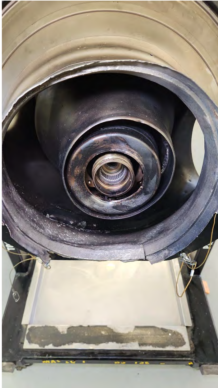
PT shaft forward looking
