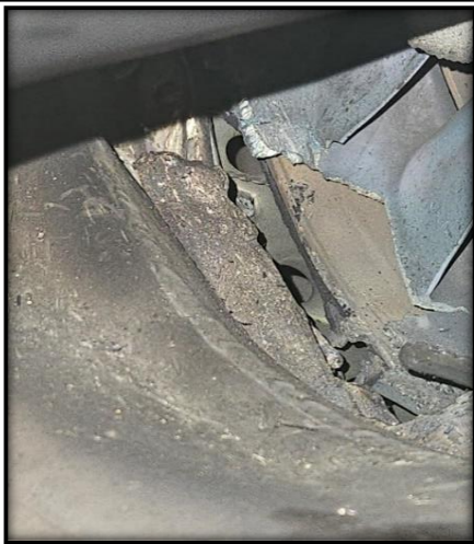
27. Damage to Exhaust Duct, PT Guide Vanes and Stator Housing.
