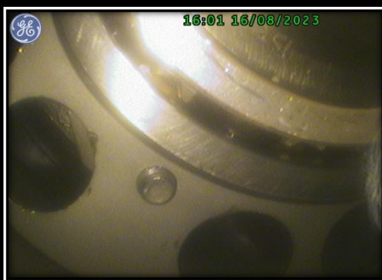
36. #4 Bearing with webbing, bolts, and bearing intact.
