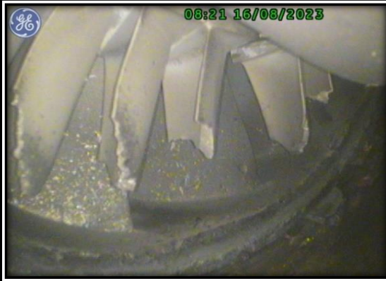
21. Power turbine blades. Heavily damaged, with breakage.
