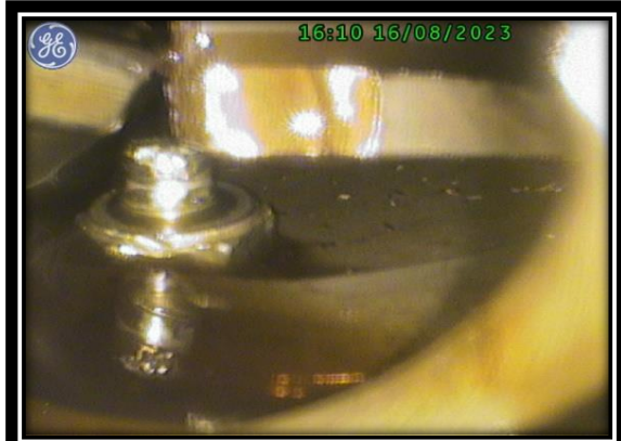
41. #3 Bearing Race Retaining Bolt, sheared.
