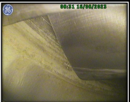
7. Signs of light rub, top of First Stage Compressor.
