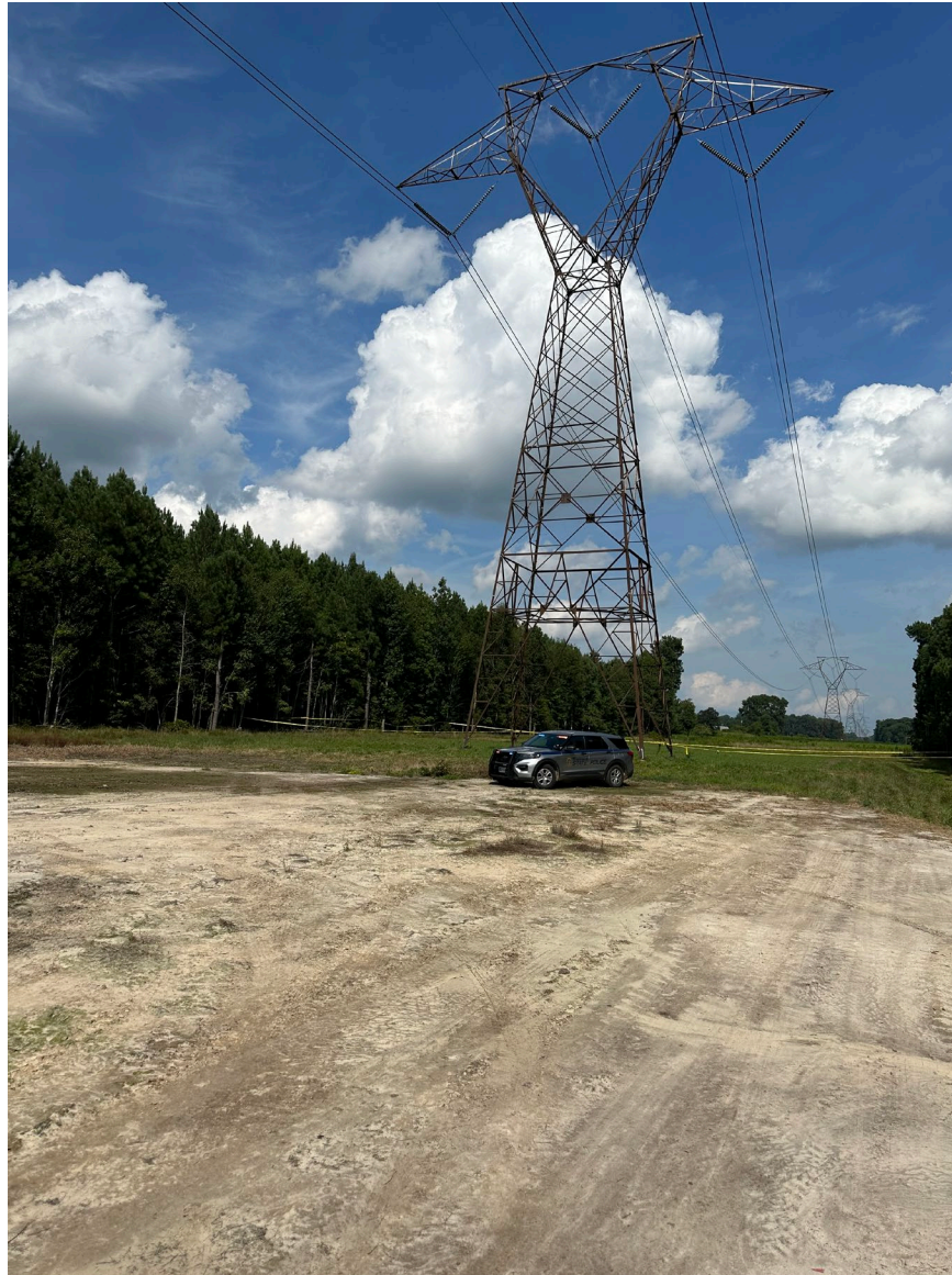
Photograph 1 - Structure (Courtesy of FAA)
