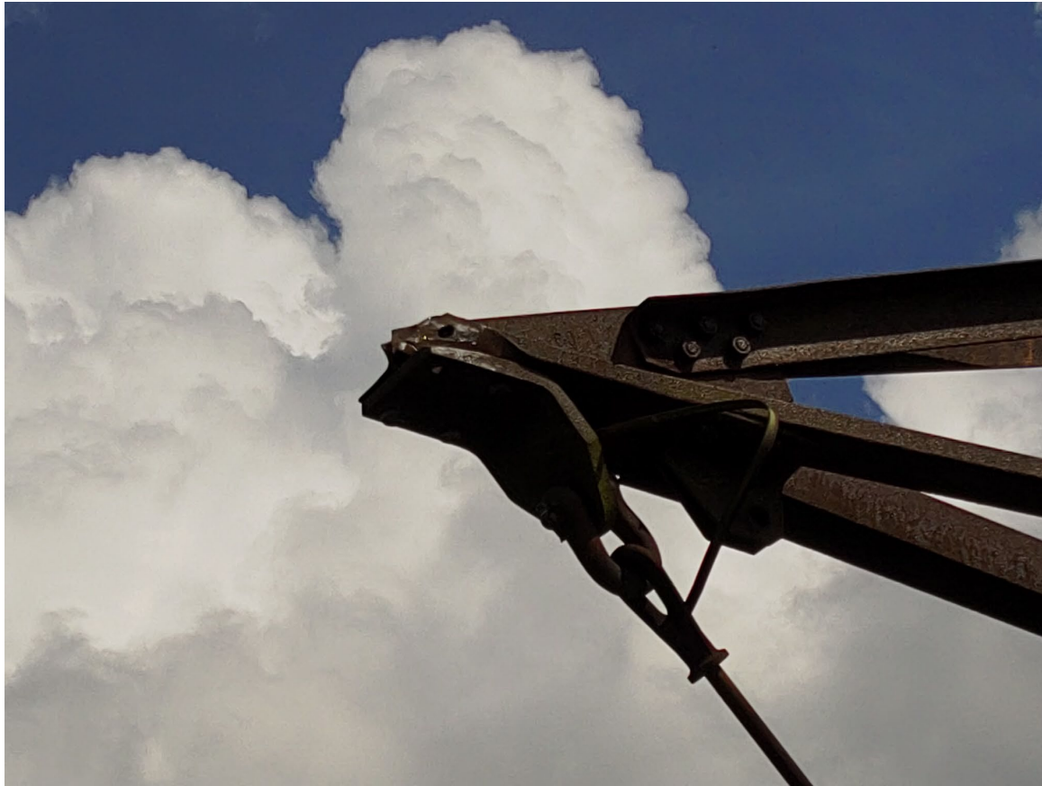
Photograph 3 - Structure Arm (Courtesy of FAA)
