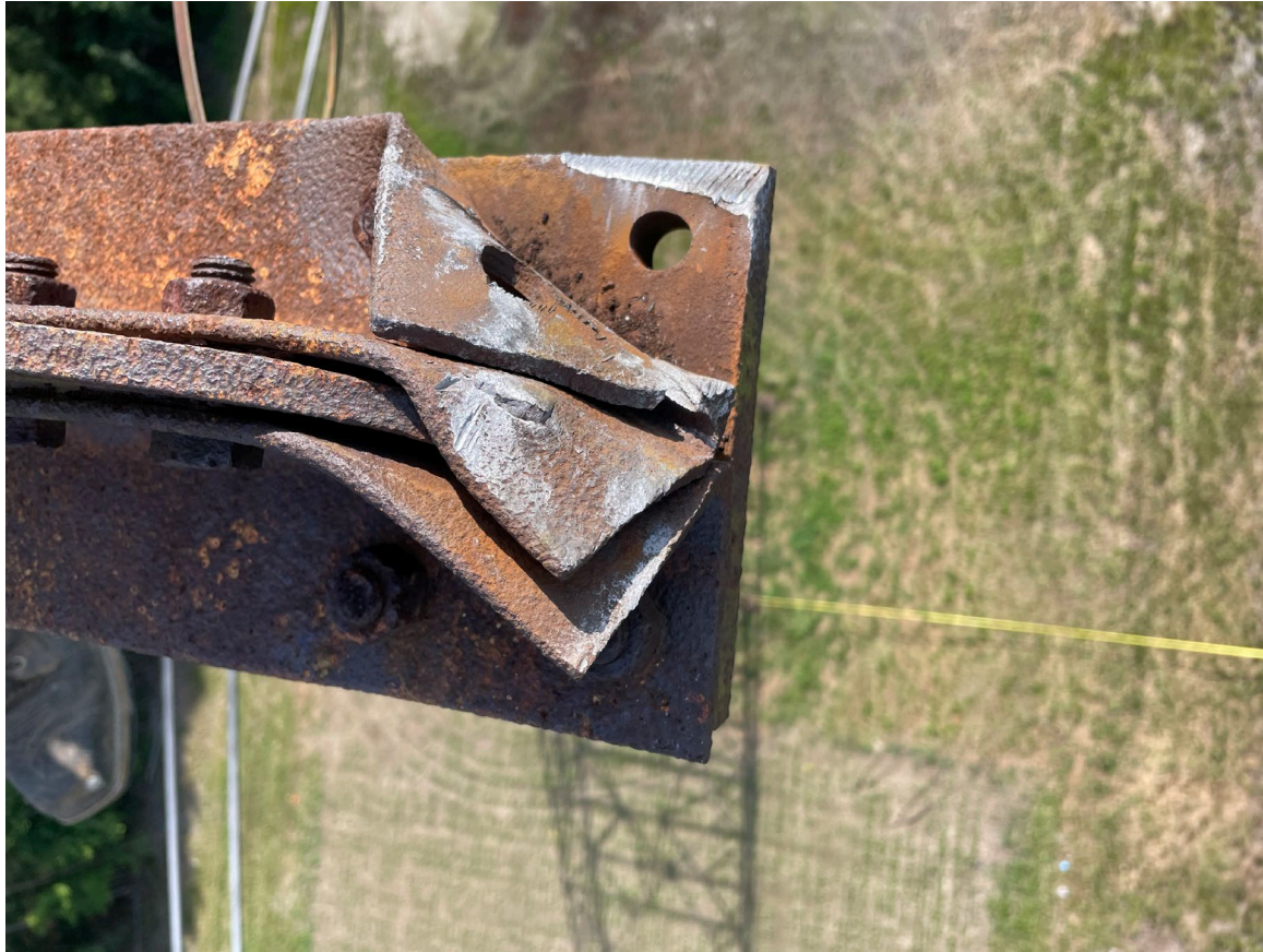
Photograph 4 - Structure Arm Close-up (Courtesy of FAA)
