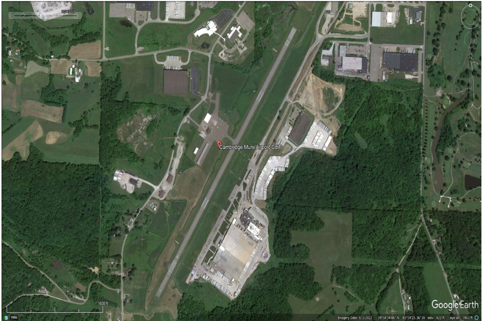
Figure A2.1: Planform view of CDI runway 4/22 configuration. The grooved asphalt pavement is 4,298 feet long by 75 feet wide. North is toward the top of the page.
