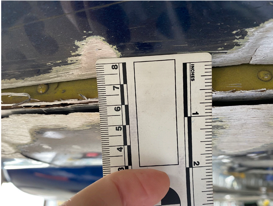
Photograph 3 - Bottom of airplane hull bucking (Courtesy of FAA)
