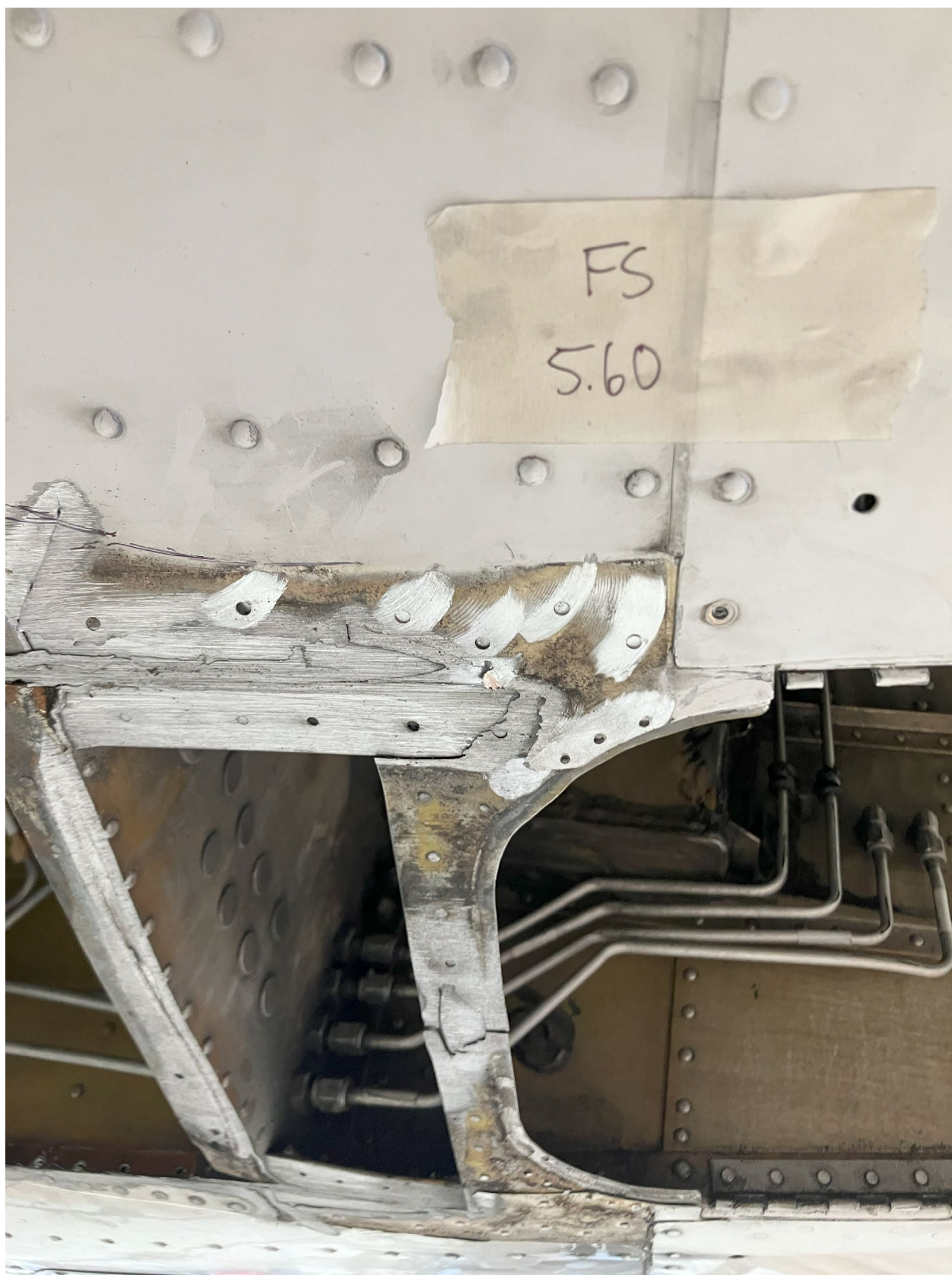
Figure 1: View looking up, FS5.5 and 12.5 (pressure bulkhead) Damaged flanges with skin removed
