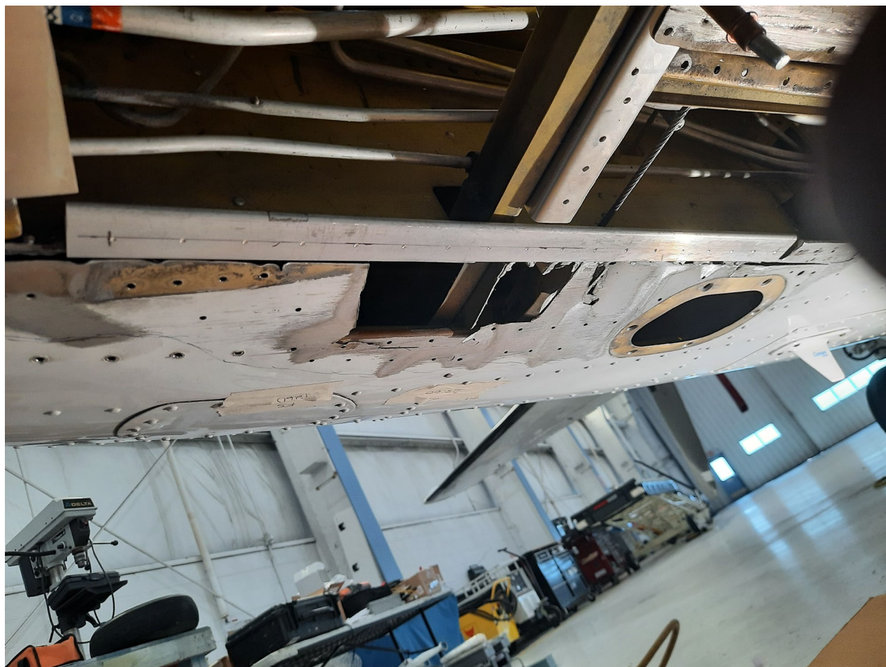
Figure 12 keelson web lower intercostals being repaired
