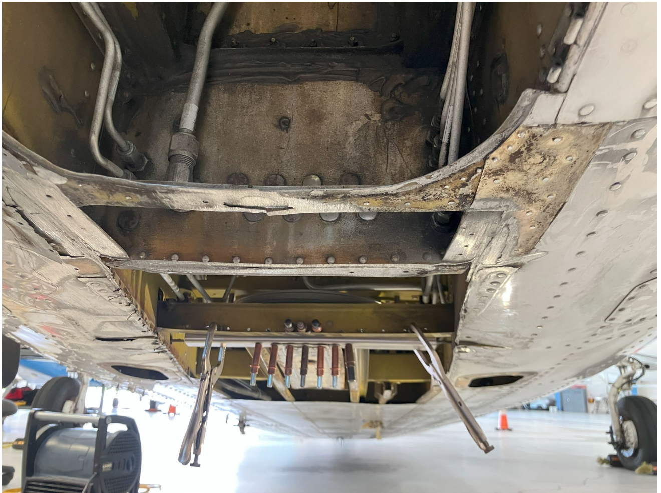
Figure 2: View looking up/aft, Repair angle at FS23.5 (fwd end of aileron drum hat channel) being worked.
