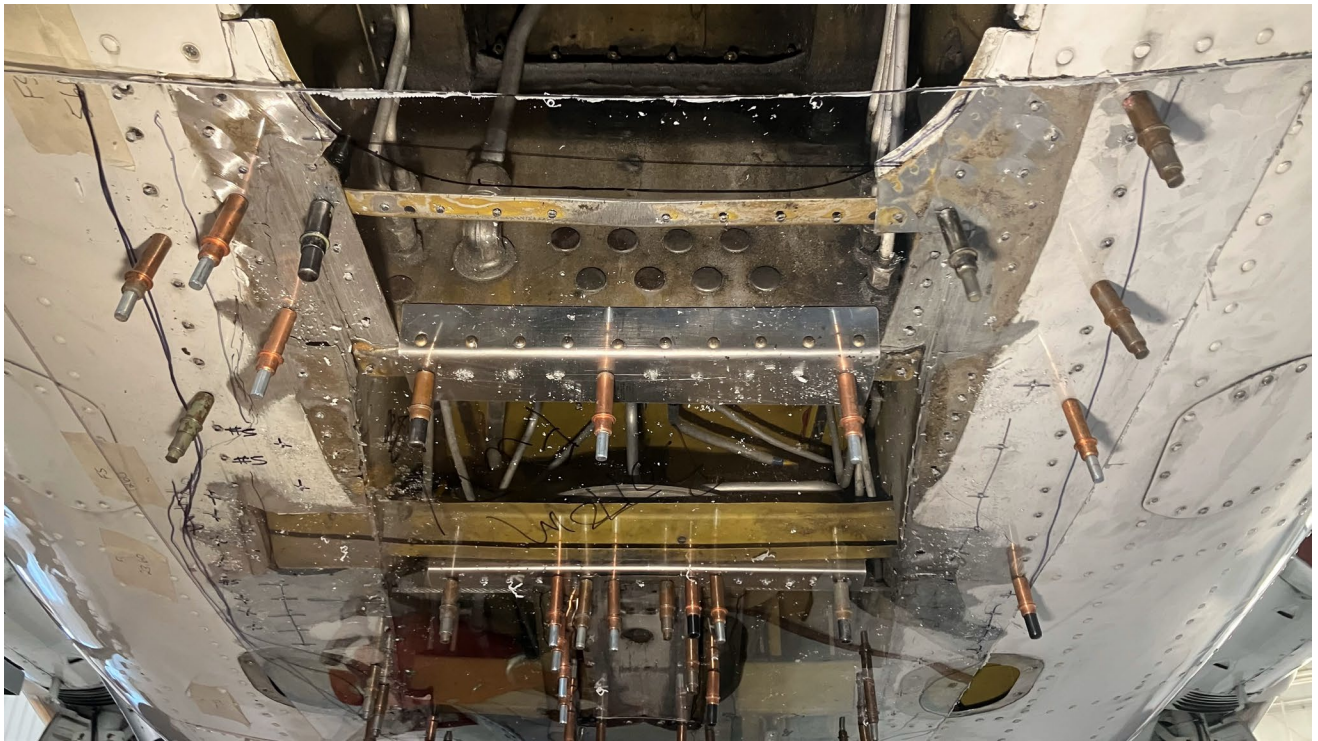
Figure 14 View looking up/aft Mylar being used to transfer holes to skin doubler.
