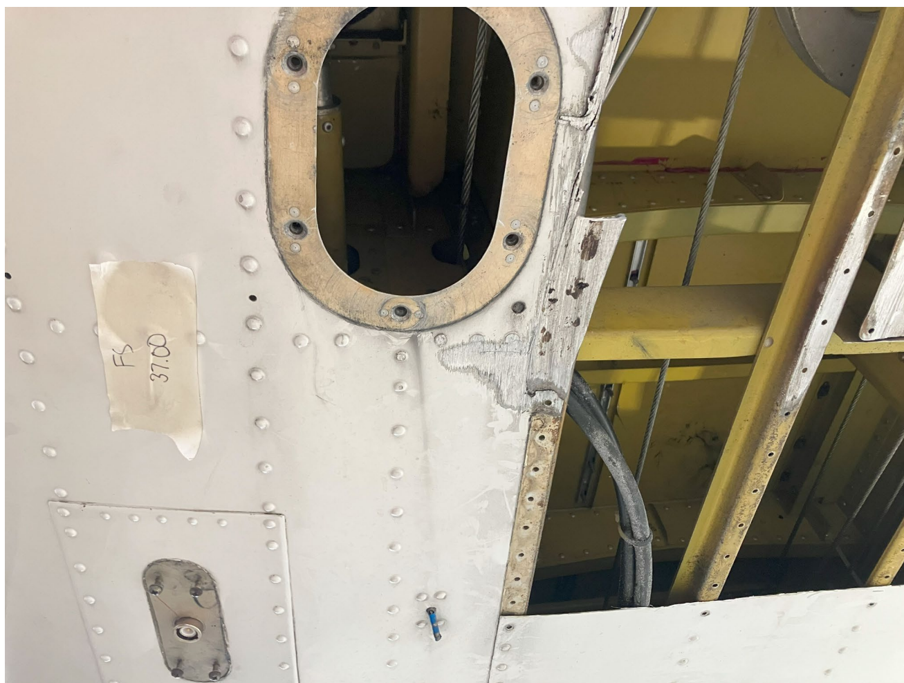
Figure 6 View looking up at FS37.0 – chafed skin cut out.
