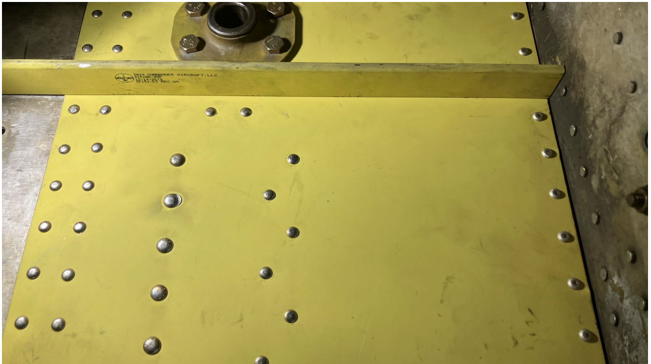
Figure 11 LH CK 159-2 being installed to keelson
