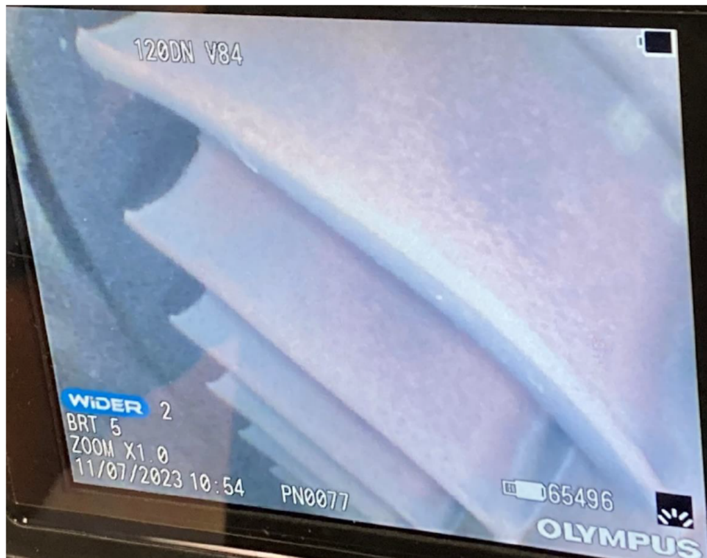
Photo No. 20, Compressor Turbine Borescope Inspection
