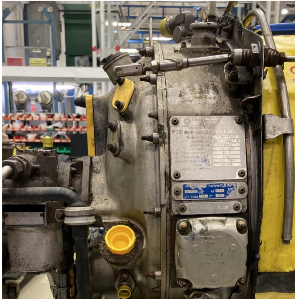
Photo No. 22, CAM Box Assembly Removed
