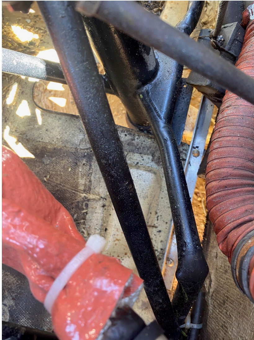
Photograph 2 - Digital Photograph From Recovery Company View of the Damaged Engine Mount
