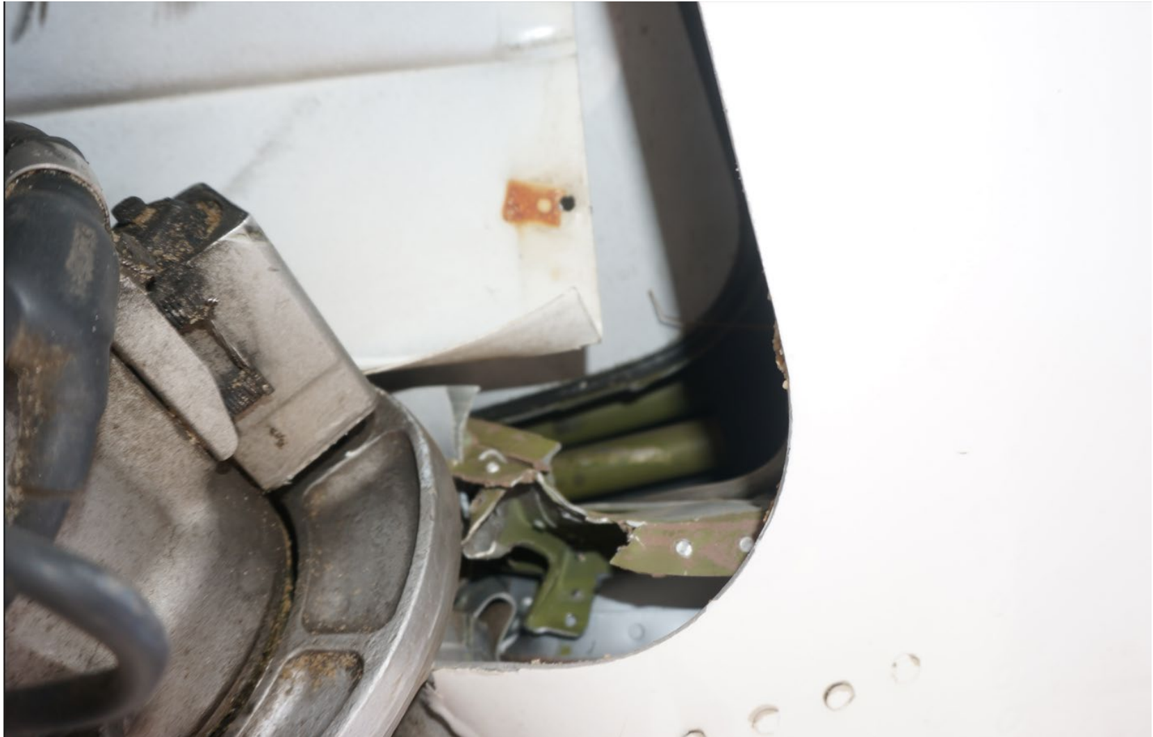
Photograph 19 - Frame 0 (Forward Pressurization Bulkhead)
