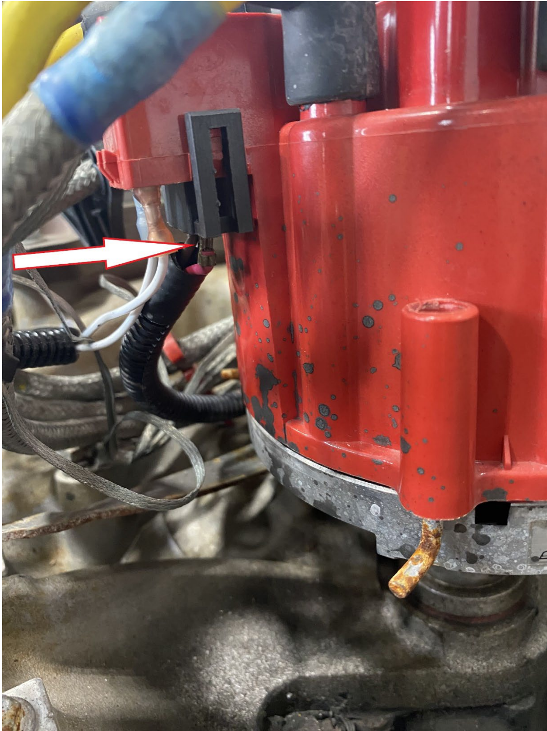
Figure 1: Annotated AMF Aviation, LLC Digital Photograph. Arrow Points to Separated Red Colored Electrical Wire at Distributor. The Wire Provides Power to the Ignition Module.
