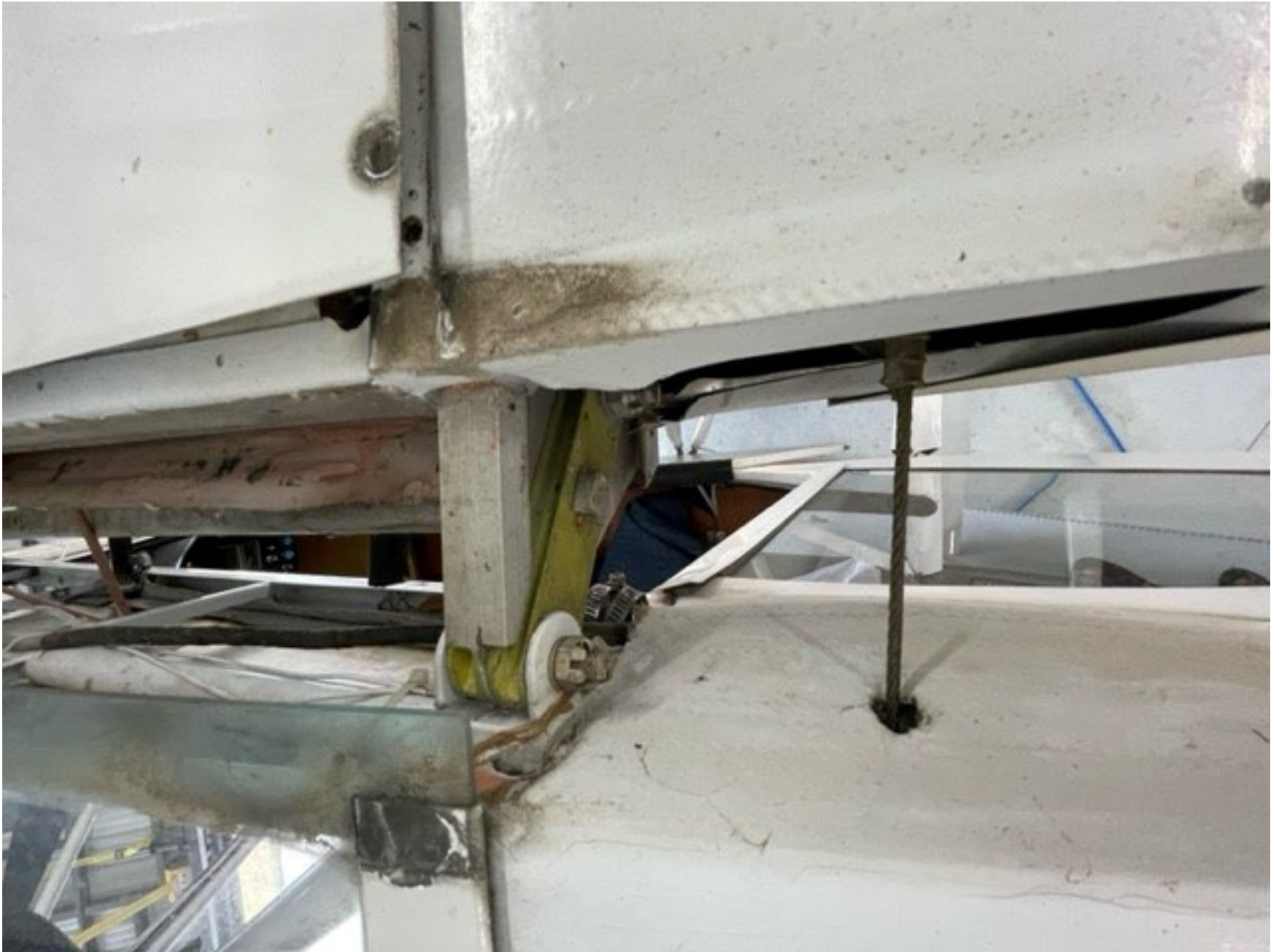
Photo 1 – View of bent wing spar (FAA Photo)
