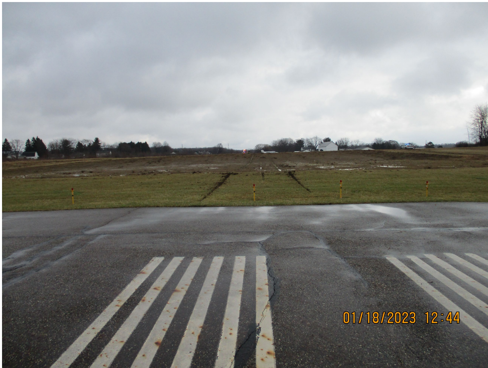
Photo 1 – View of Runway Departure End, Ground Tracks, Berm, and Airplane at Rest Where Found (FAA)
