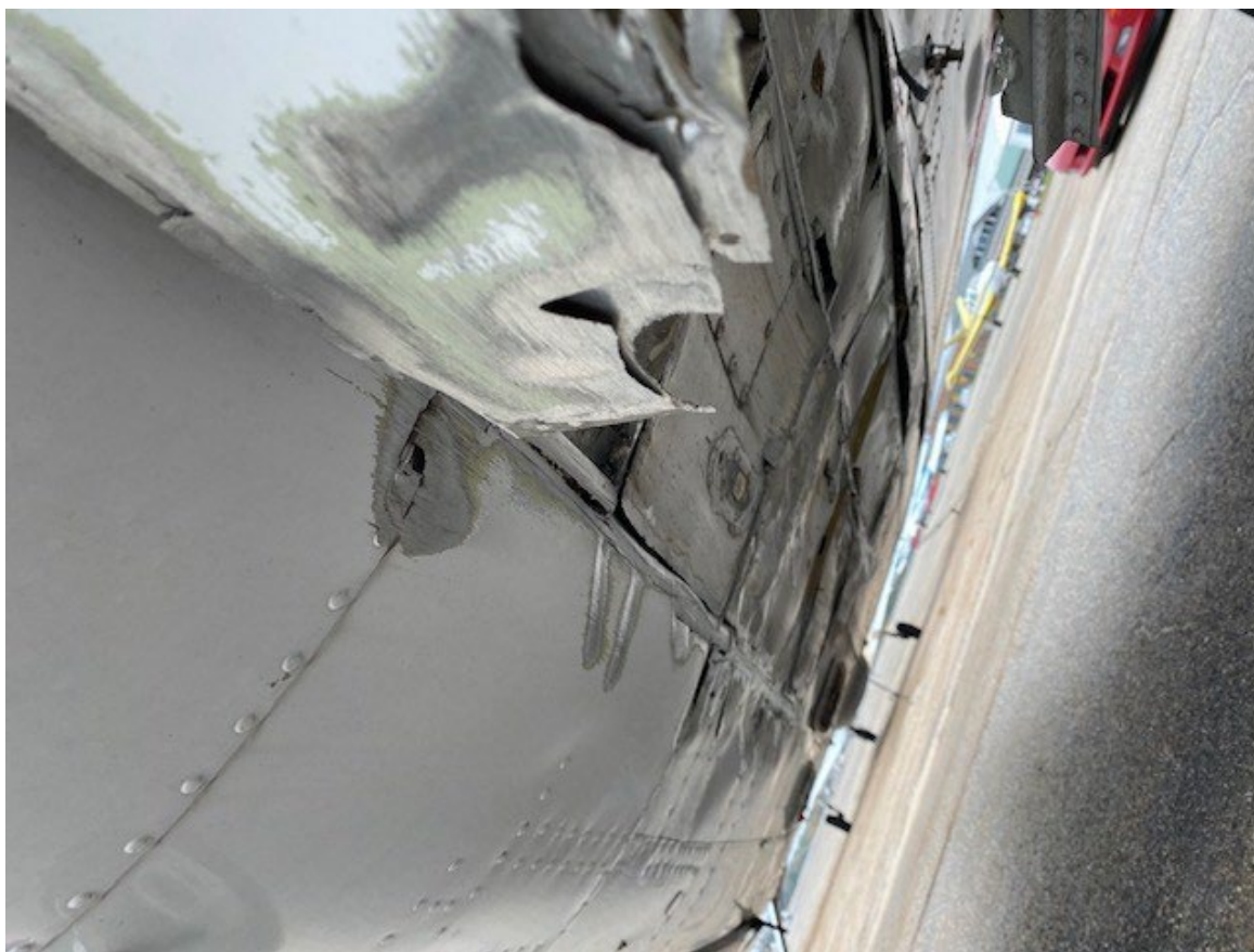
Photograph 1 - Lower Fuselage Skin and Structure Damage (Courtesy of FAA)
