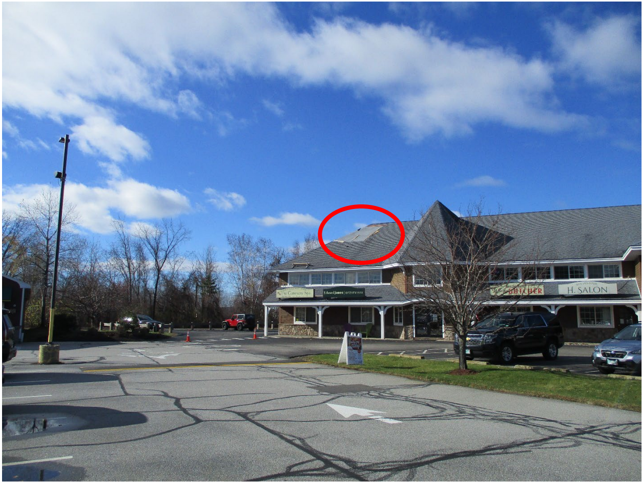
Photograph 2 – Building damage [red circle] from airplane impact
