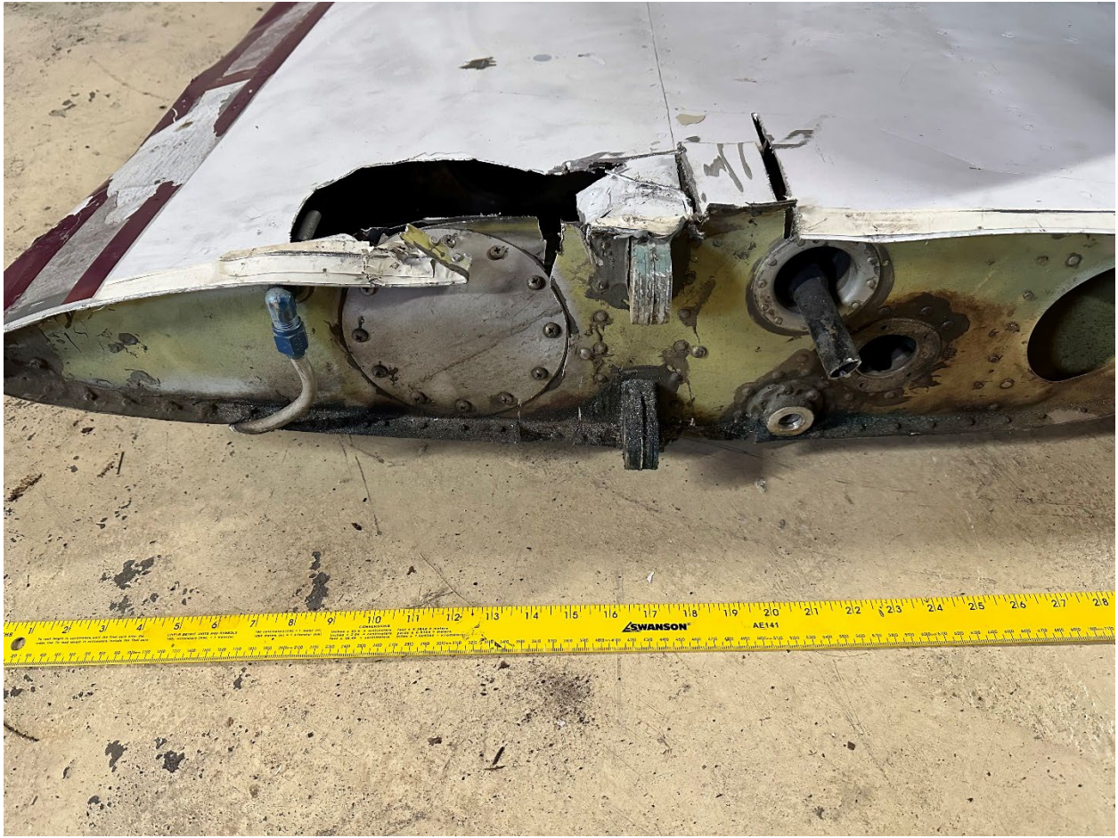
Figure 1: Digital Photograph from SE Avionics. Photograph IMG_9299. View Depicting the Wing Root of the Right Wing. Note the Sealed fuel fitting Boss and other sealed openings in the Inboard Rib aft of the Main Spar. This is consistent with a fuel tank aft of the Main Spar.
